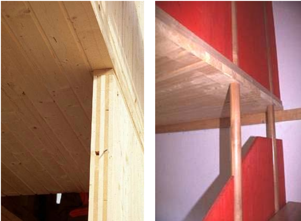
Figure 6 Massive timber plates: Diaphragm action and plate action allows for new architectural timber-based expressions and multi-functionality in a single element.
