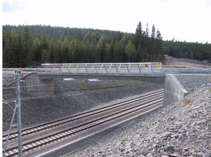
Figure 5 A SCC bridge over a railway outside Motala, Sweden.
